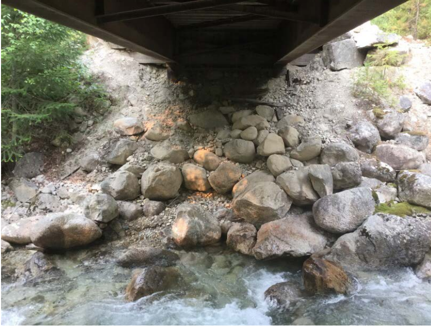
Right Bank Abutment when facing downstream
