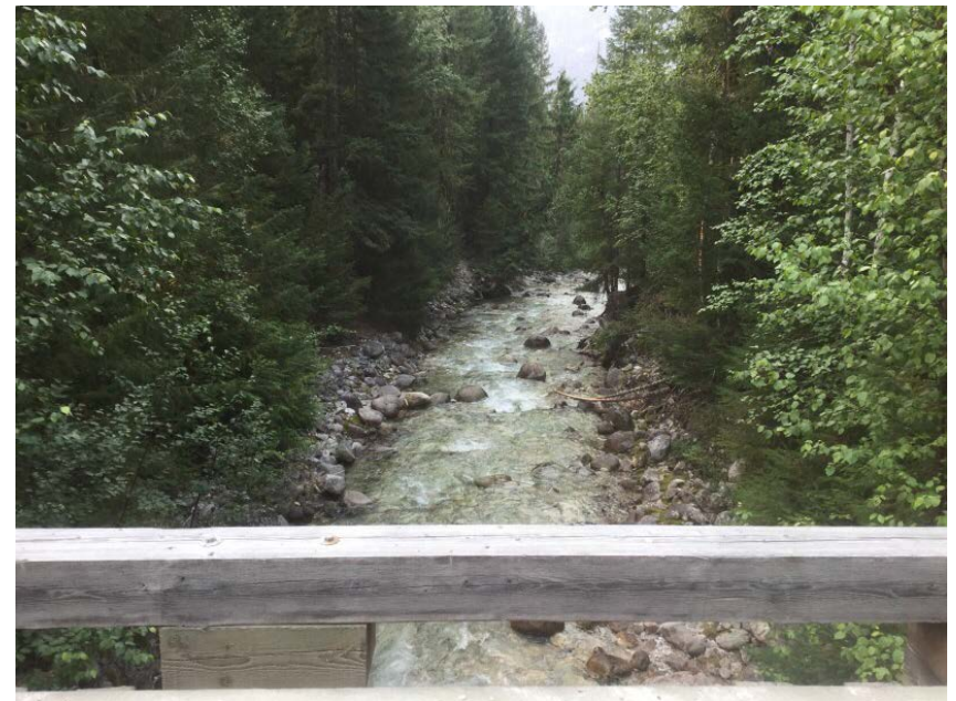
Looking downstream from deck
