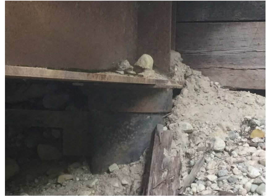
Upstream right bank bearing, typical all 4 corners
