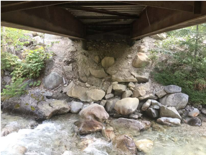
Left Bank Abutment when facing downstream
